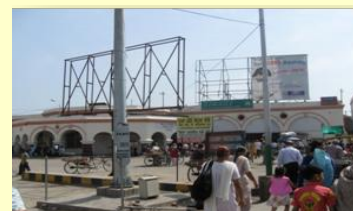
FIG. 64 RAILWAY STATION SOURCE: (PUDA, 2010)
