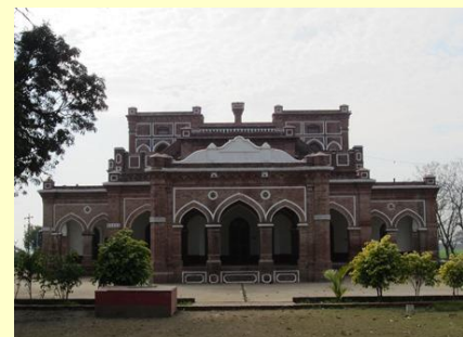
FIG. 70 VIEW OF HAVELI AT BAGHRIAN (SANGRUR)
